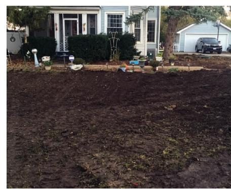
The completed MBR installation shows only a few riser lids peeping above grade. Notice the restricted space to the left and right of the home. The backyard was similarly small, necessitating placement of the drainfield in the front yard.
