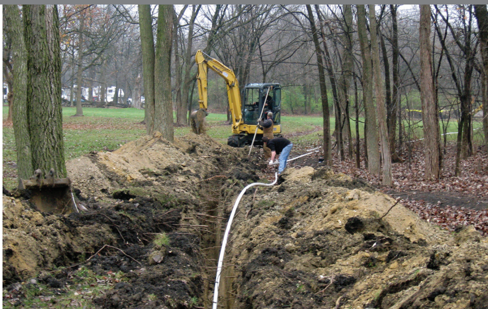
Matt Moser (foreground) and Ben Hoffman lay 550 feet of 1.5-inch PVC Schedule 40 low-pressure pipe as Jim Koltunchik uses a Komatsu excavator with 12-inch bucket to trench from a holding tank to the septic tank. (Photos courtesy of Zeiter's Septics Unlimited, Morris, Ill.)
