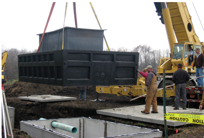
Workers prepare to set the bottom half of the aerobic treatment unit in its concrete tank.
